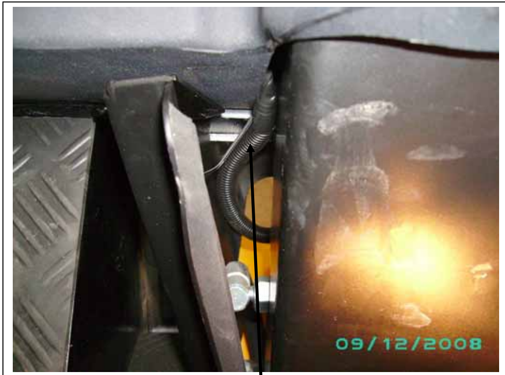
Electrical going to relay from fuse panel shown at floor of cab.
